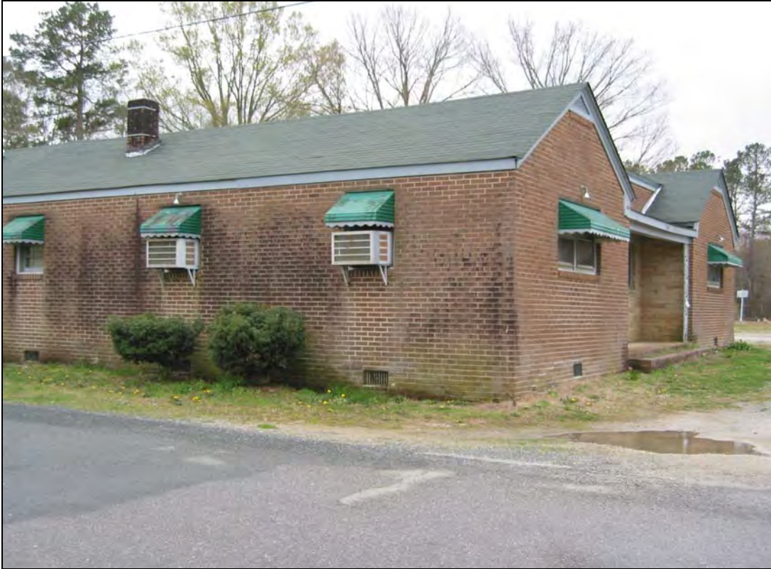
Above: VIP Club, northeast corner (2008)
