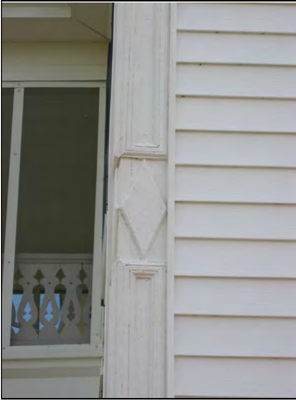
Above and below: Jernigan House, cornerboard detail
