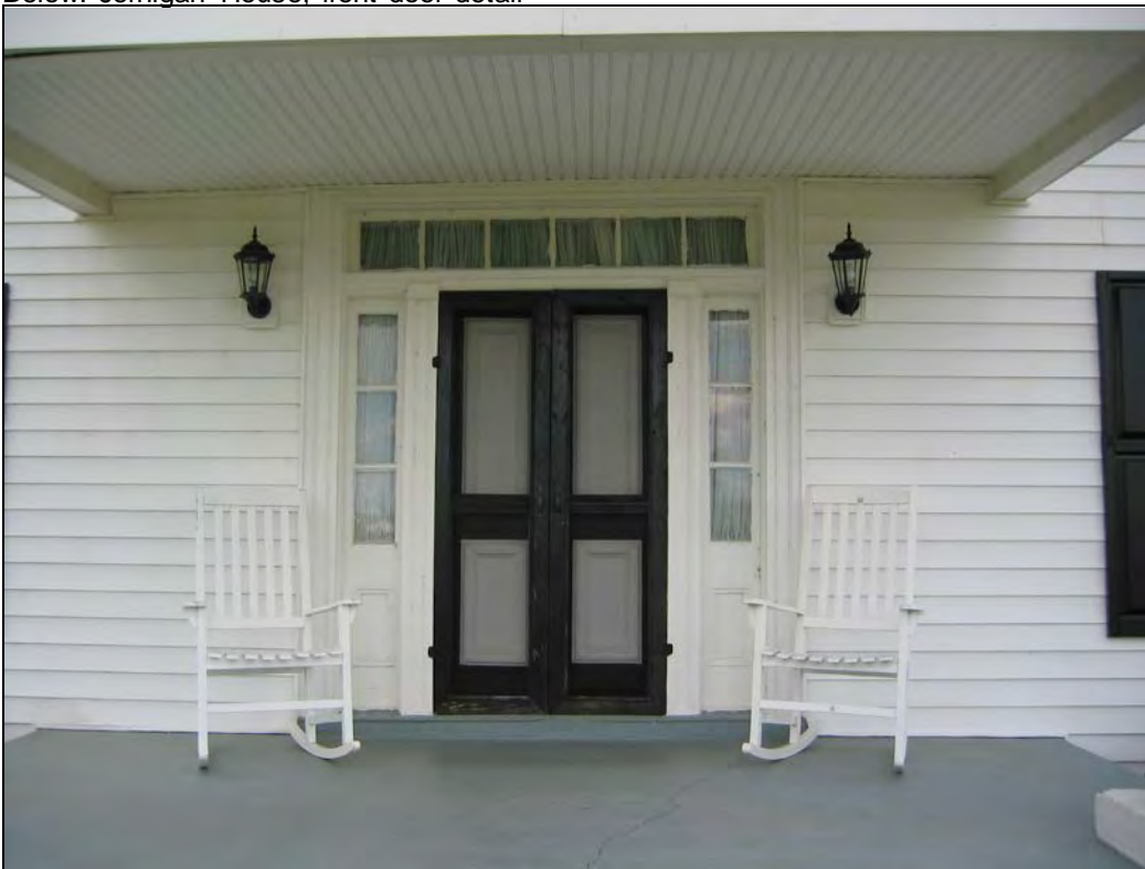
Below: Jernigan House, front door detail
