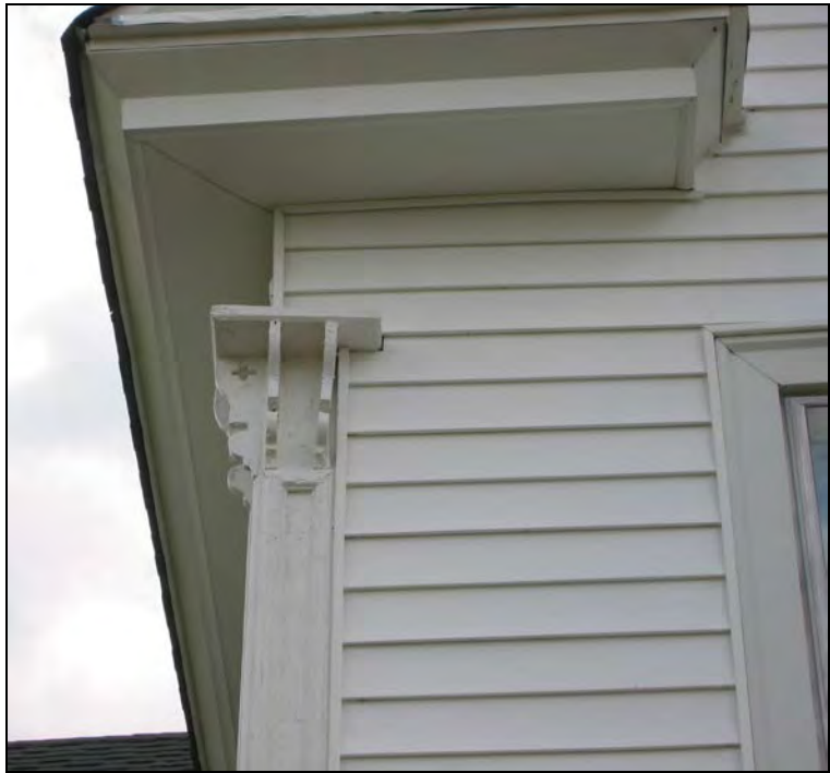
Above and below: Jernigan House, cornerboard detail
